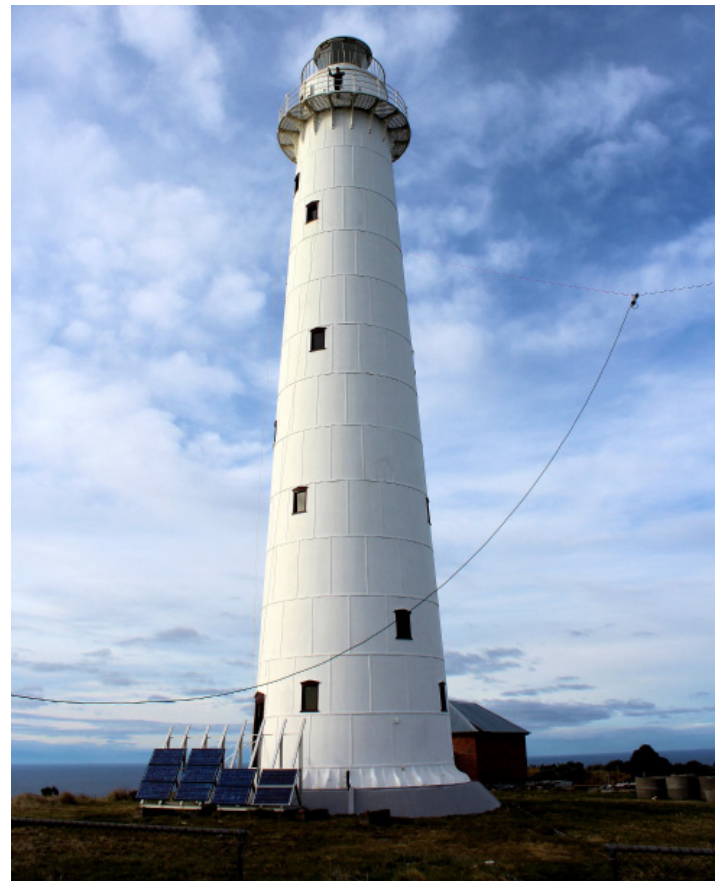
The aerial rigged up from the lighthouse to Quarters 3
